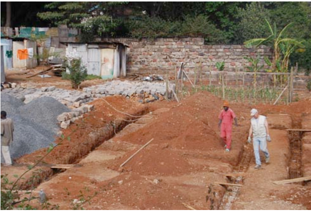
The foundation is dug...by hand
