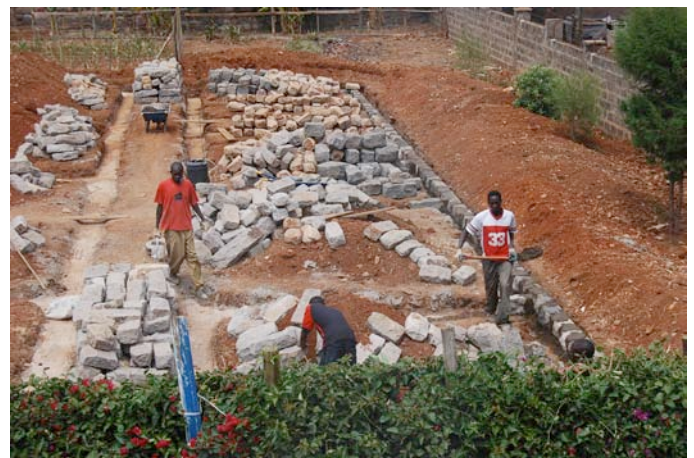
The foundation blocks are placed
